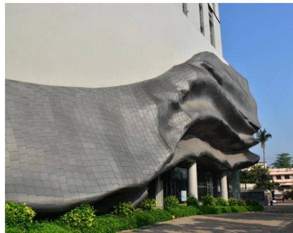
Esplanade One Mall, Bhubaneswar (Inde) Agence d'architecture : Practice Design Pvt. Ltd Crédit photo : VMZINC - © Vikash Choudhary
